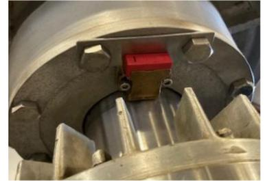
BPK-SB installed on a pump motor
